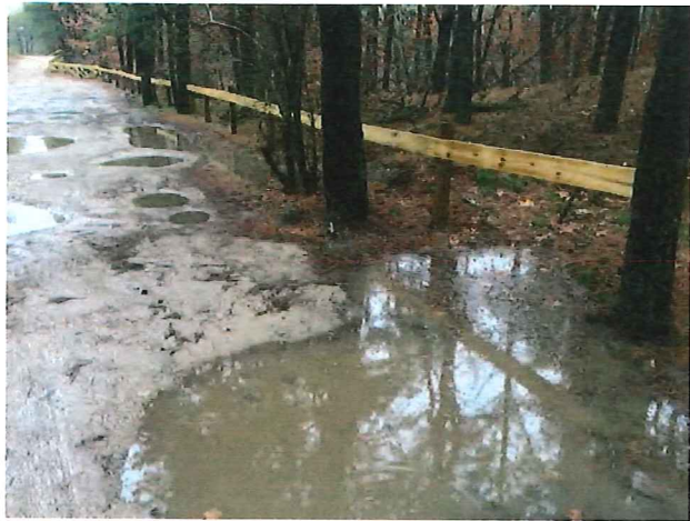
62 - Very deep pothole & drainage problem on E side of road slightly N of south end of fence (which is in the road layout), potholes
