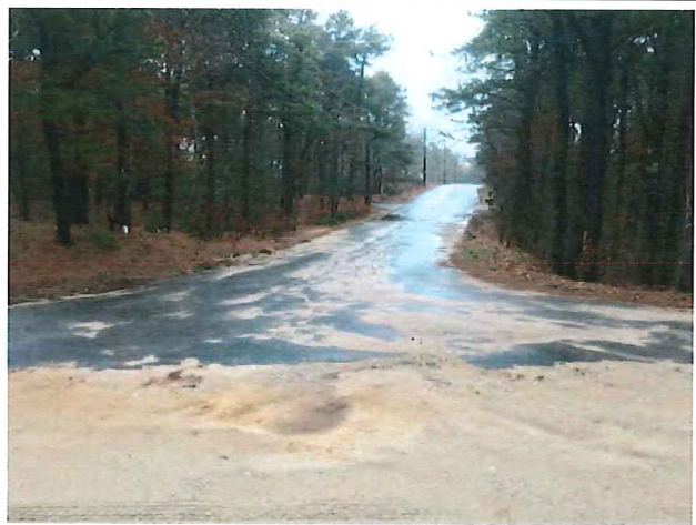
32 - Looking E down Woodland Way from intersection w/ Hay, potholes @ end of pavement
