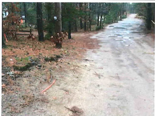
55 - To avoid the huge pothole in the road, drivers have been driving onto the shoulder of the road, exposing telecommunications line (see tire tracks around exposed line) which was formerly buried at least 24"
