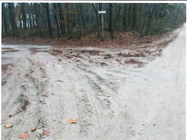
21 - Very soft sand @ end of Uncle Nates Way where it meets Hay- deep ruts
