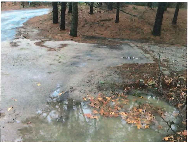
44 - Drainage problem @ SE corner of DP/Hay intersection, another view
