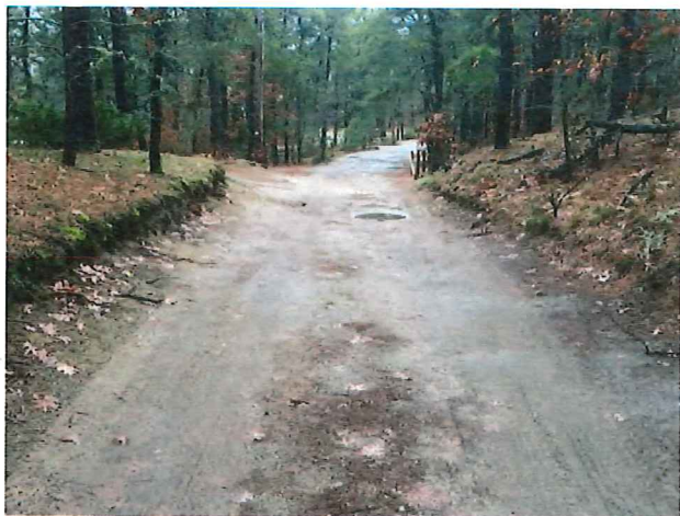
53 - Looking NNW up Hay from N of DP/Hay intersection, potholes, high shoulders on both sides of road
