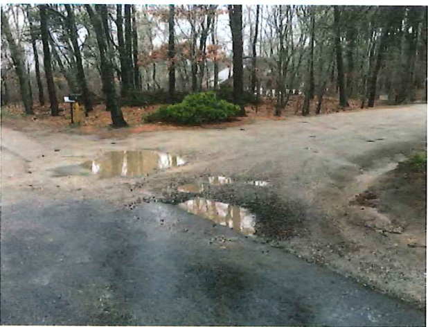
4 - Potholes on S end of dirt section of Hay @ intersection w/ Gov P
