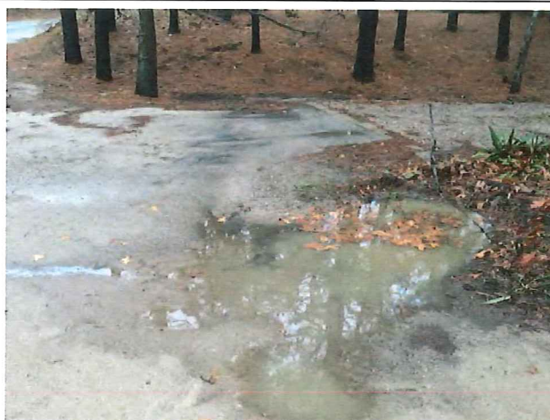
43 - Drainage problem @ SE corner of DP/Hay intersection, another view
