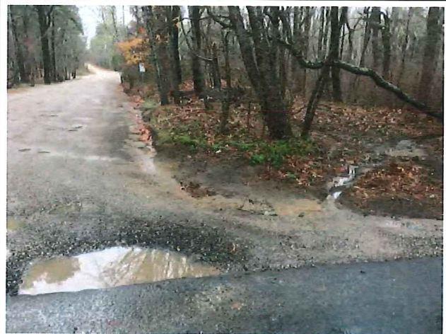
3 - Potholes on S end of dirt section of Hay @ intersection w/ Gov P, draining on R into wetland on E side of Hay (Eastham Conservation Foundation)
