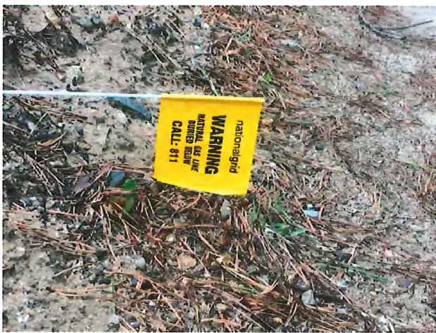
92 - Flag marking underground gas line along west side of road in front of Parcel 14-236 (1670 Bridge Road), vulnerable to damage from vehicles?
